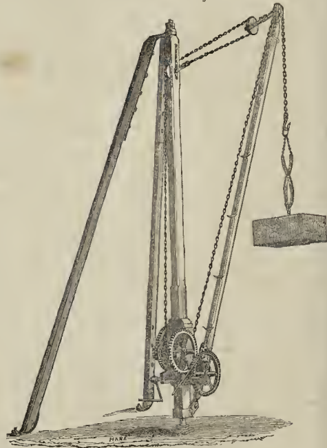
Derrick crane used at Granton Pier (Edinburgh).
